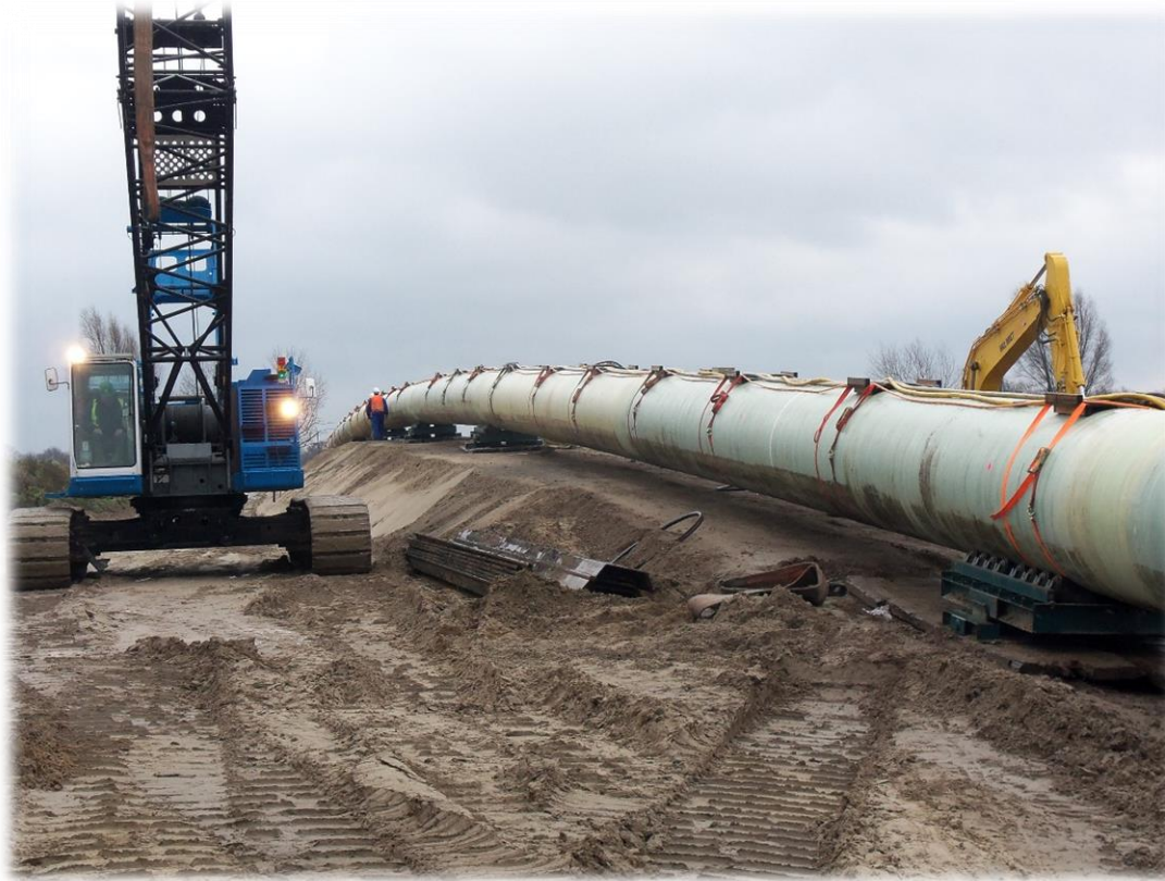
ELBE River Crossing (NEL Pipeline) – 2011 – 1078 m x 56" - HDD
