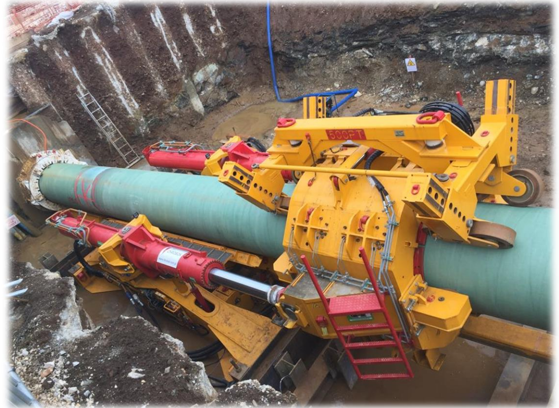
Aliakmonas River Crossing (TAP Pipeline) – 2018 – 540 m + 600 m x 48" – Direct Pipe®
